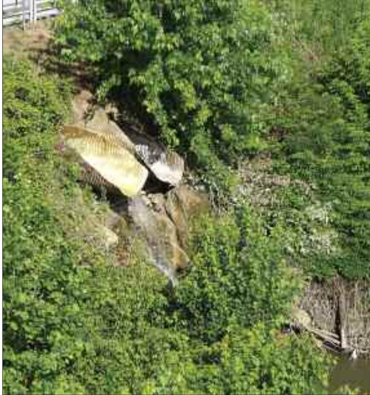
**The foreground pipe is shown lined and is back in service while the other pipe has had its flow diverted while being prepared for lining. The pipes discharge directly to the Susquehanna River.**
