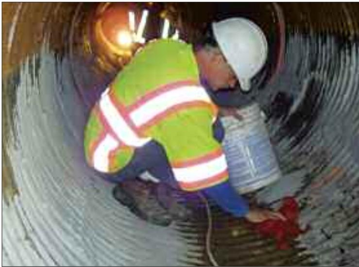
**Charlie Mitzel, spray application technician, uses absorbent material to remove water from between the corrugations in the culvert before final drying of the pipe.**
